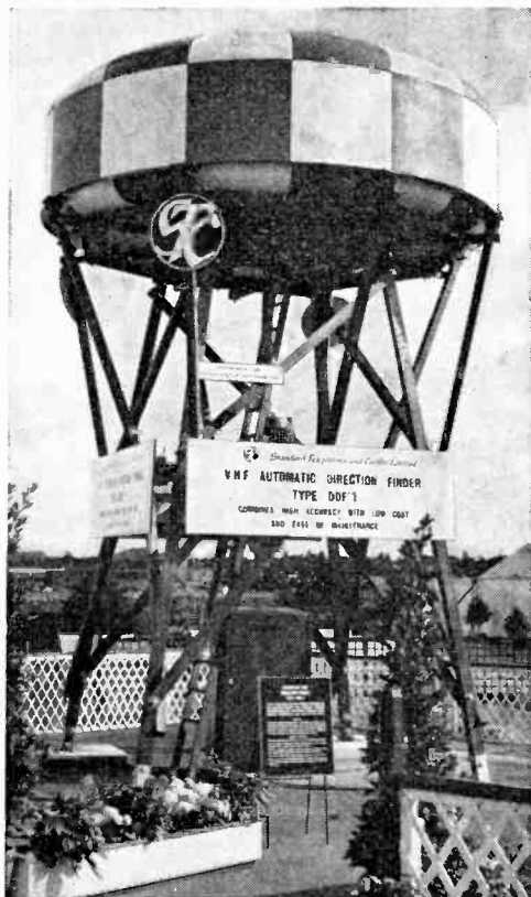
The long-base S.T.C. Doppler direction-finder aerial. The only building required is the wooden scaffolding, as the Doppler signal and reference signal are fed by land-line to the indicator.
